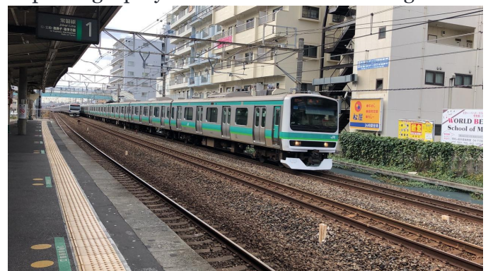
Two JR East express trains pass each other at Minami-Kashiwa station near Tokyo on January 4, 2020. Commuter and intercity trains play a critical role in transportation in Japan.
