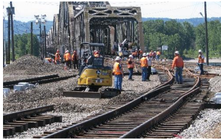
BNSF rebuilds the junction in Vancouver, WA in April 2015. Major track changes here will speed freight and passenger train movements.
