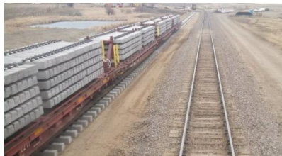
Second main track construction west of Minot.
