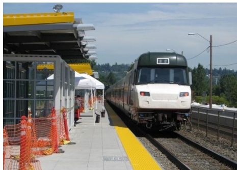
Cascades 500 departs the under-construction Tukwila Station on July 12, 2014.
